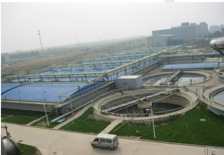
华药大型污水处理厂异味收集装置 Large-scale sewage treatment plant for chemicals--- odor gathering devices
