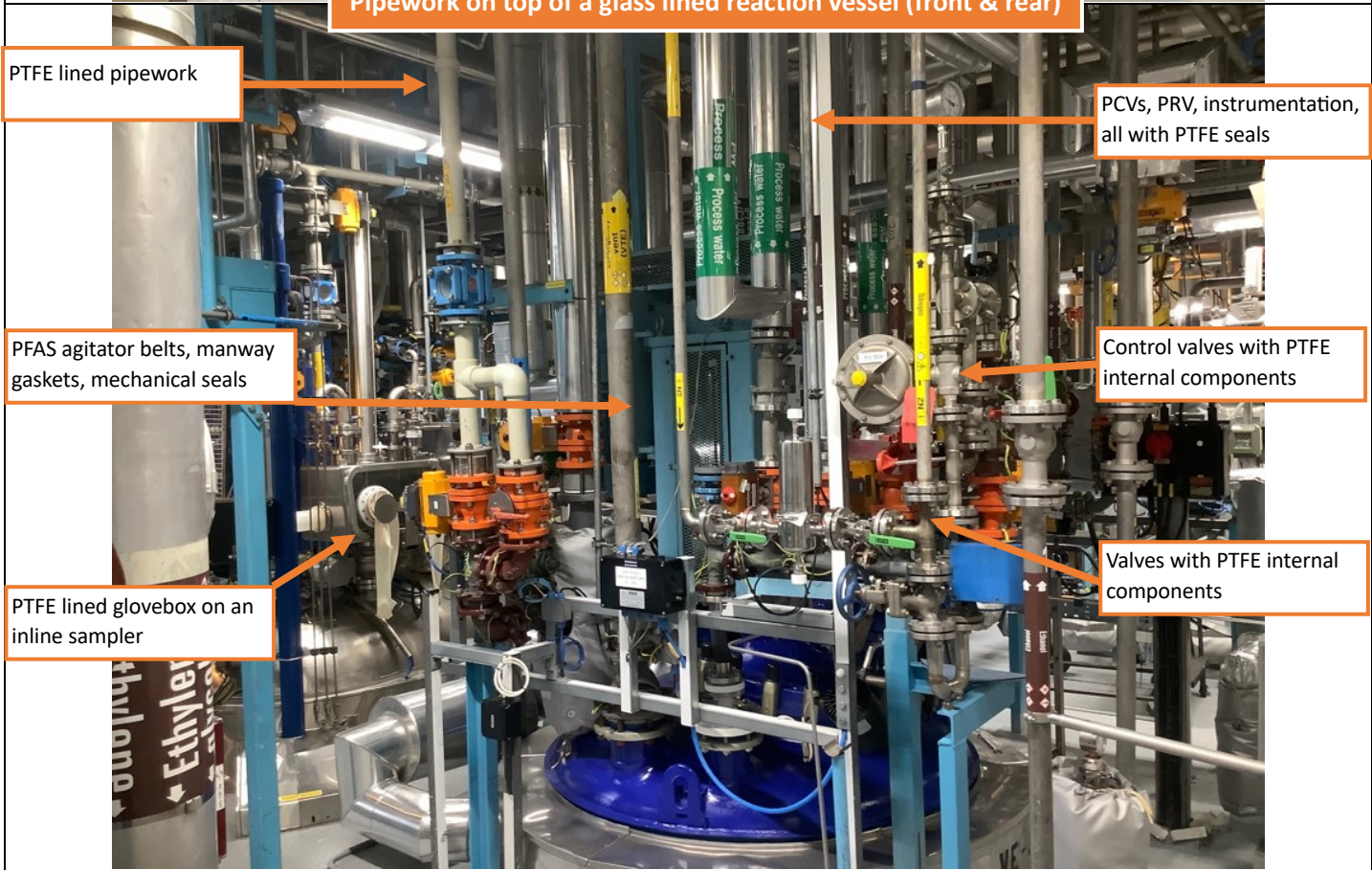
Pipework on top of a glass lined reaction vessel (front & rear)
